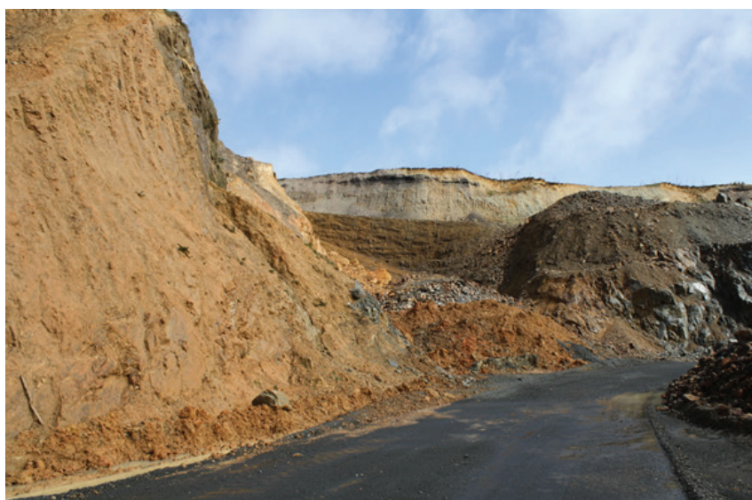
Figure 5 - Haul roads must be clear of spillage.
