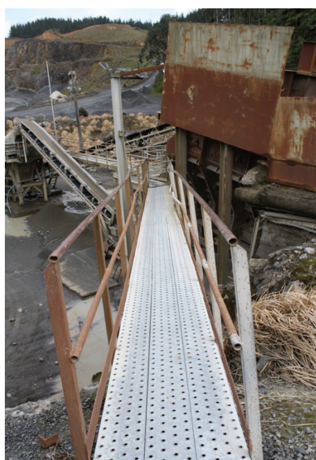
Figure 8 - A clear raised walkway
